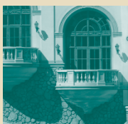
Figure 1. The front porch of this house is more than 40 inches from the ground. Therefore, it requires a ma'akeh of at least 40 inches high.
